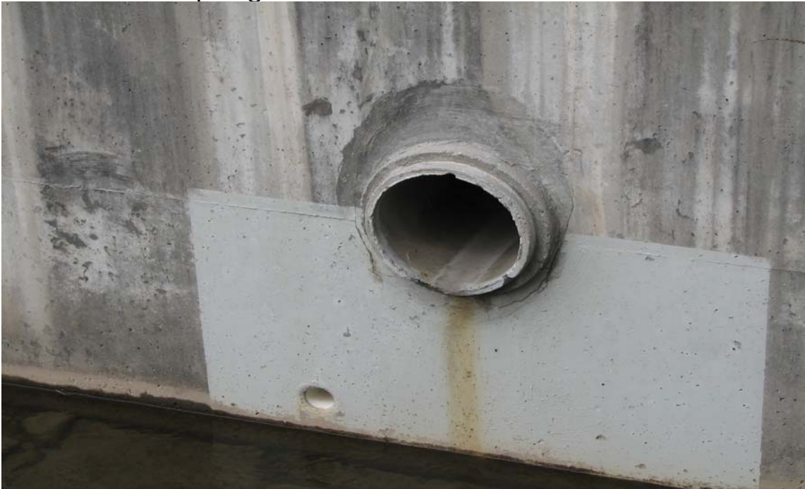
Outfall on Mill Run - Normal (dry weather, no flow).
