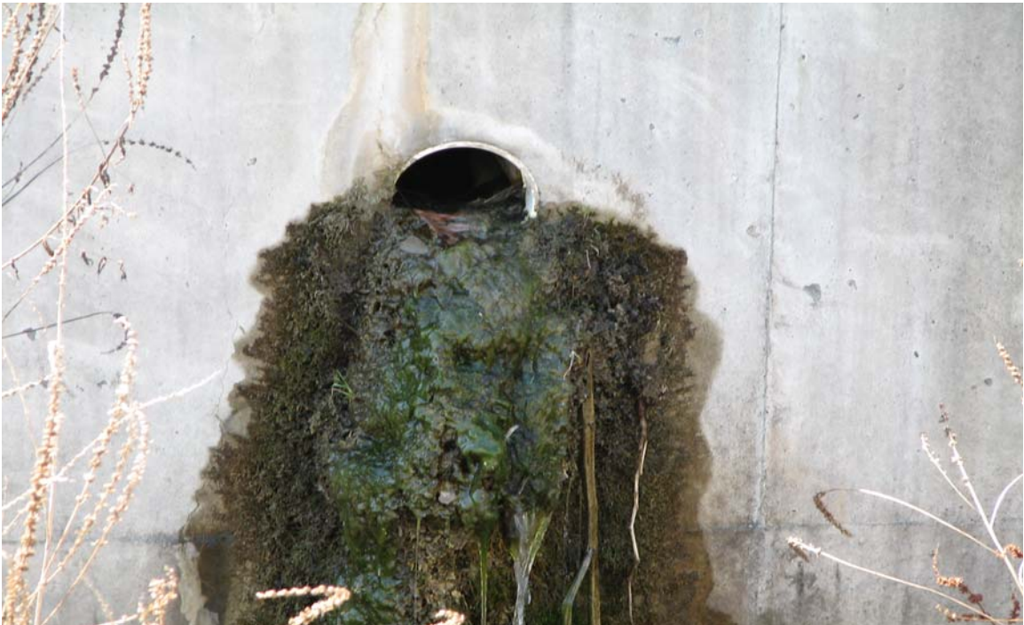
This is an outfall that you would CALL on... any flow in dry weather (48 hours without rain) especially if something unusual is going on with its discharge.
